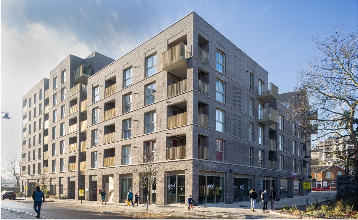
BLOCK D – TRINITY PLACE, YORK ROAD
